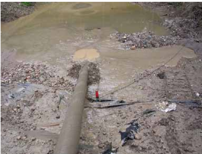
Exit of the bore at the aiming dowel after 1600 meters.
