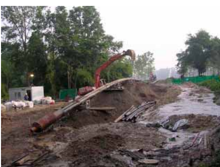
Top bend construction during pipe pulling.
