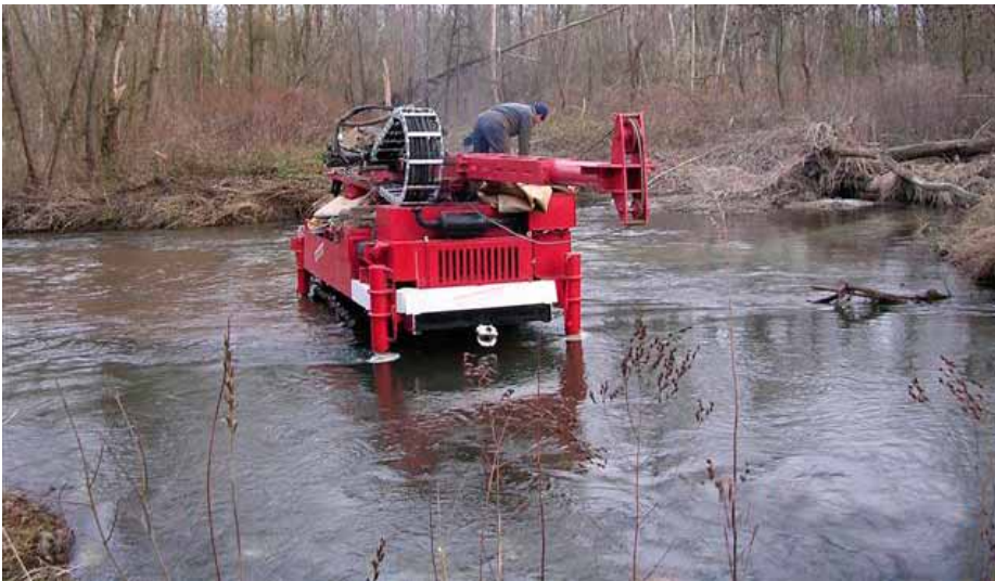
Soil investigation bore in the river.
